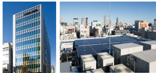
Case example: Photovoltaic facilities installed on the roof of a building
